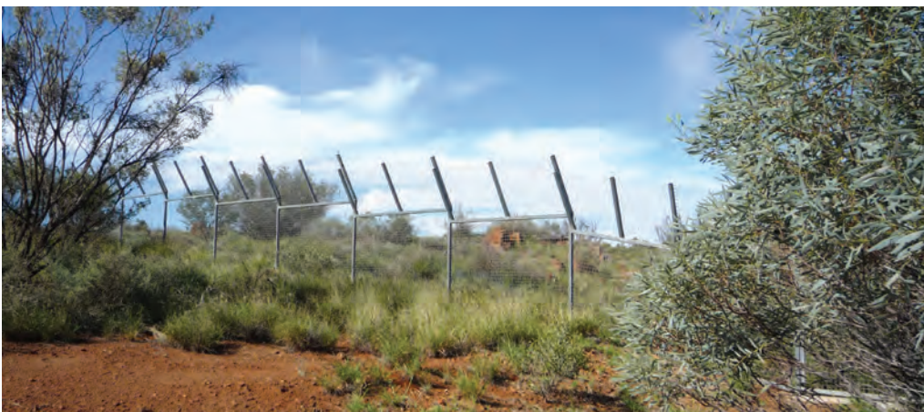
Perimeter fence at TPN
