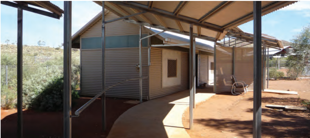
Sheltered path to bedroom unit at TPN
